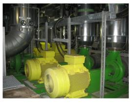
The Unterhaching was the first geothermal power station in South Germany. It makes use of the Kalina system ( $\sim 11\%$  water, 89% ammonia) as the working fluid (boiling temperature of mixture is  $50^{\circ}$ C). It was initially planned for electricity generation, but the main focus shifted to district heating since, after 18 months, due
